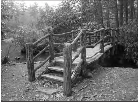
Rustic Bridge at Highlands.
